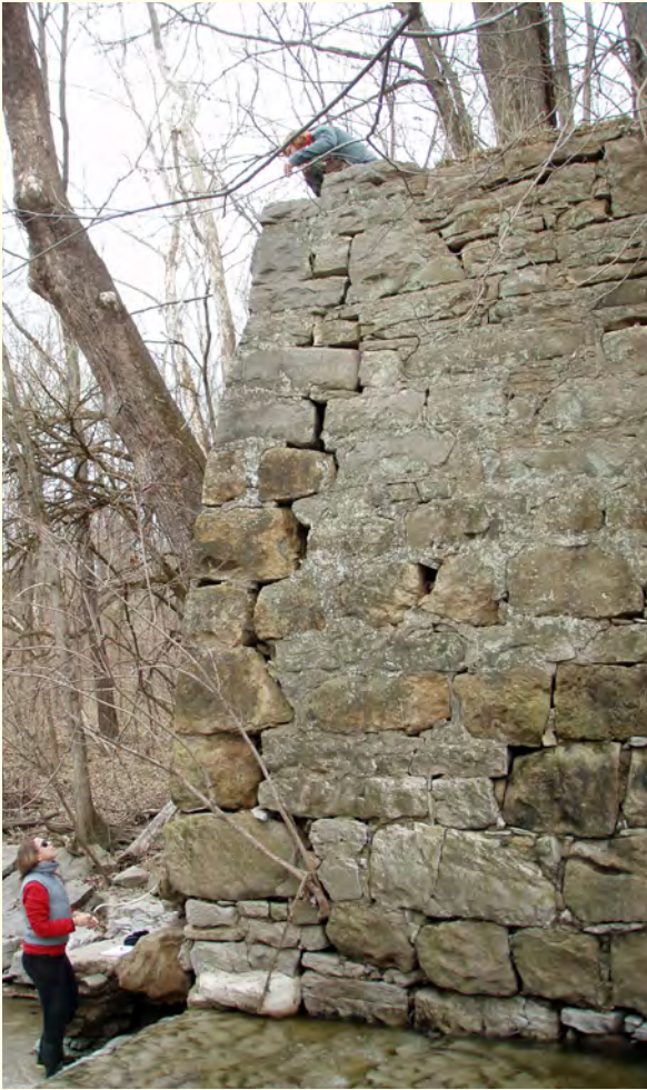
Lindley bridge remains, mid-Nineteenth Century, Little Piasa Creek, Madison County.
