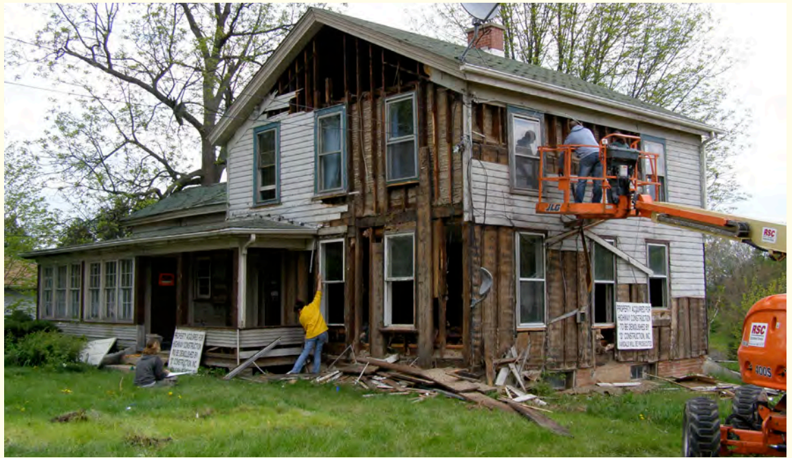
Stripping siding from 1830s timber frame residence, Yorkville.
