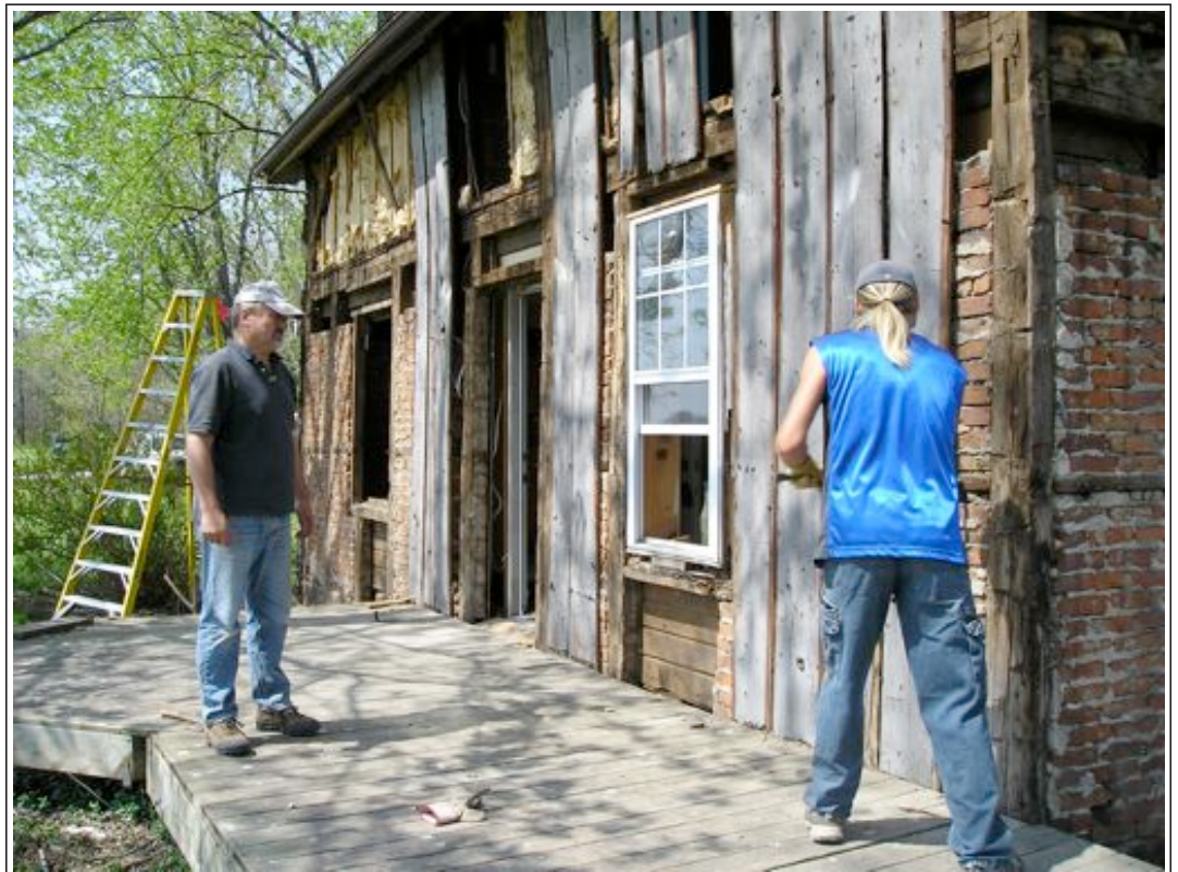
DeBaun House, pre-1840 hand-hewn, timber-framed structure, Madison County.
