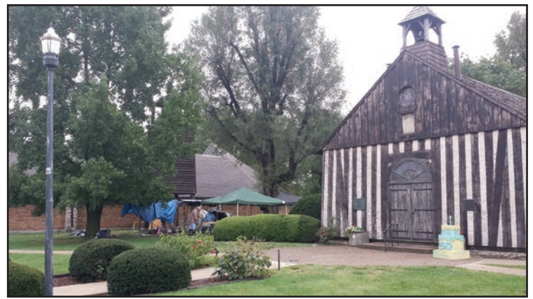
The Holy Family Church site with excavations in the background.
