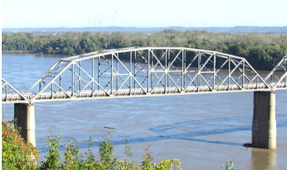
Figure 12: The main channel span of the Champ Clark Bridge, facing northeast
