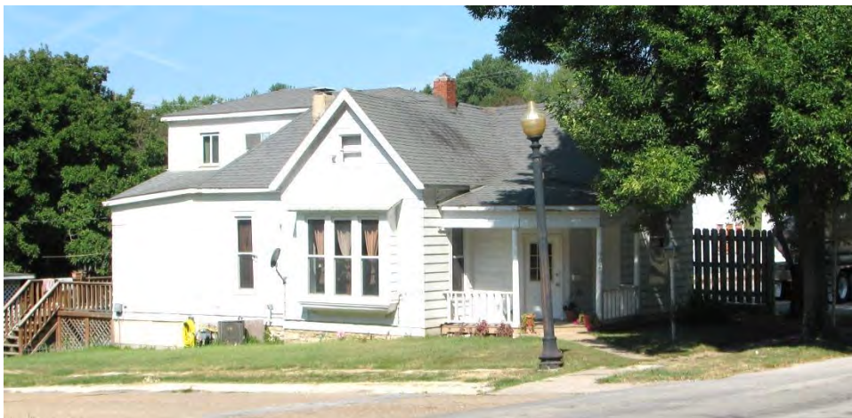
Figure 15: Architectural Resource 24, facing northwest
