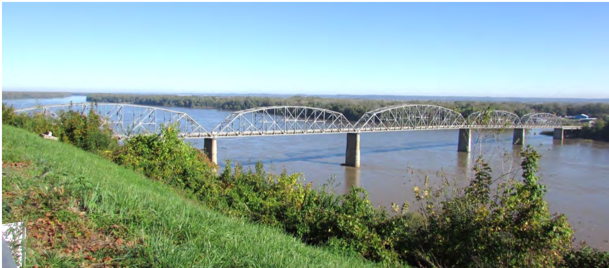
Figure 11: Champ Clark Bridge, facing northeast
