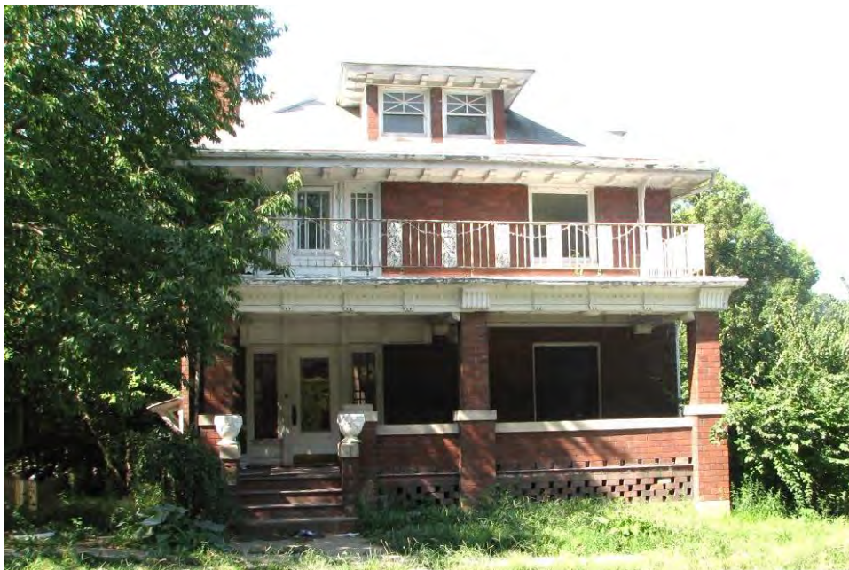
Figure 16: Architectural Resource 25, facing west
