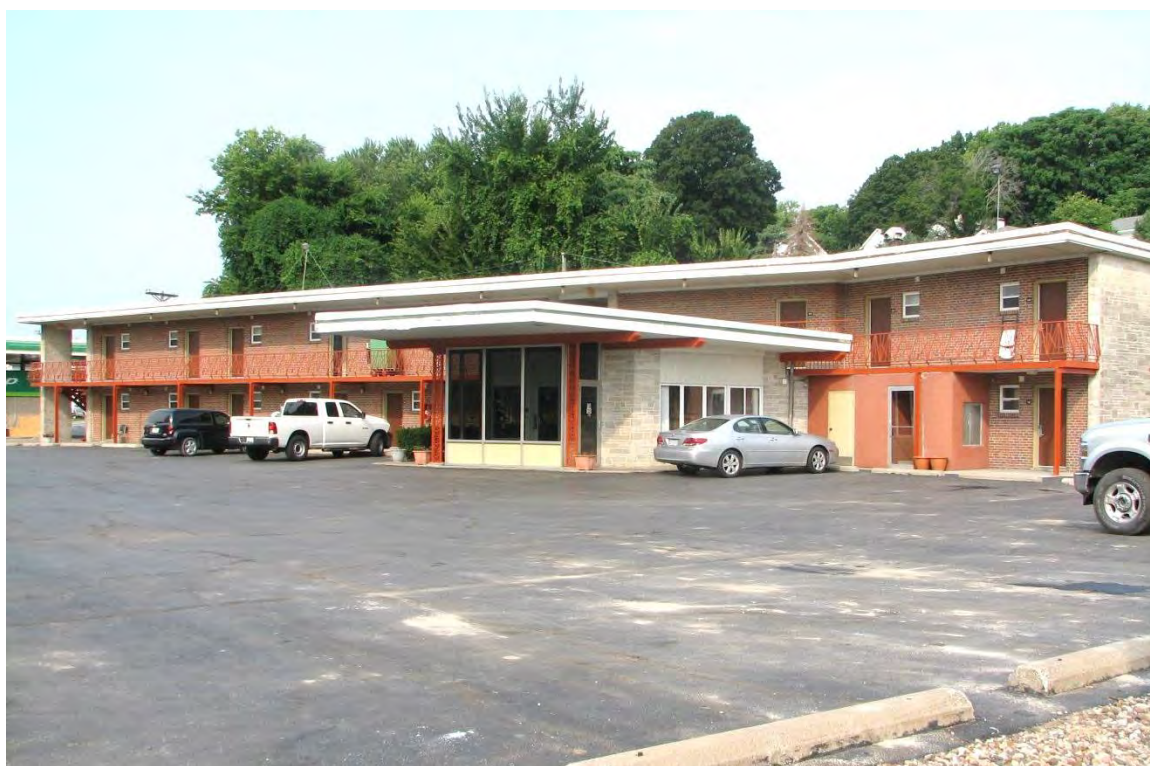
Figure 3: Architectural Resource 4, facing northwest
