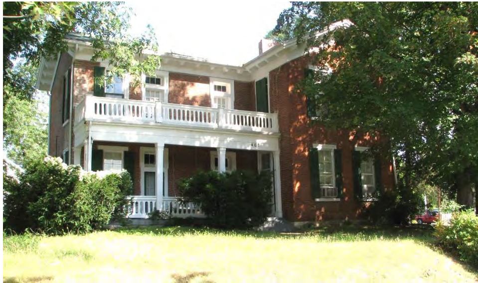
Figure 9: Architectural Resource 41, facing northeast
